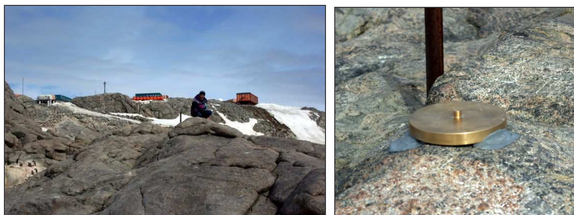
Figure 6: Installation du repère N
